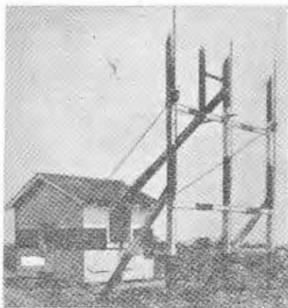
Fig. 3.—The aerial system of a 33 Mc. radio range as used in Australia. These aeri- als are placed at the top of towers approx. 90 feet high.
