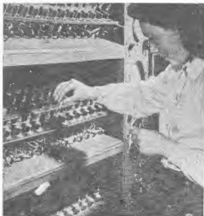
After the sub-miniature has been pumped, it is processed before testing. This breaking-in stage is carried out in banks of 60.
