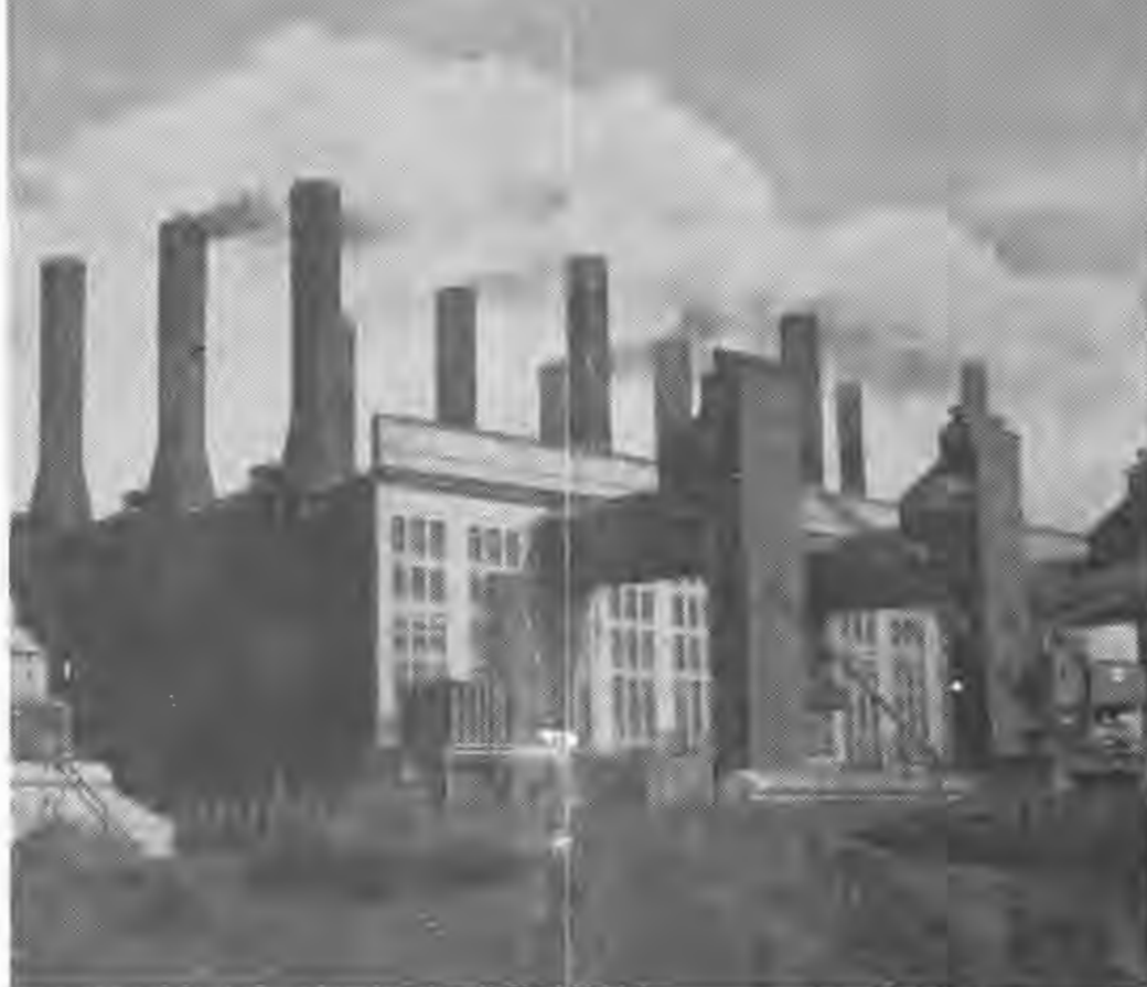
A general view of the Power House.
