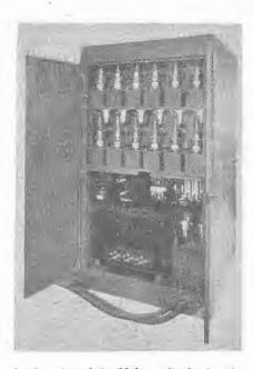
Another view of the 20 kw. unit, showing the twelve mercury vapour rectifier valves high tension transformer and other power control components.
