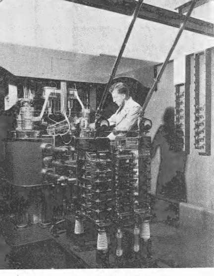
The Australian designed 100 kw. r-f power amplifier installed at Shepparton. RADIO SCIENCE, April, 1948
