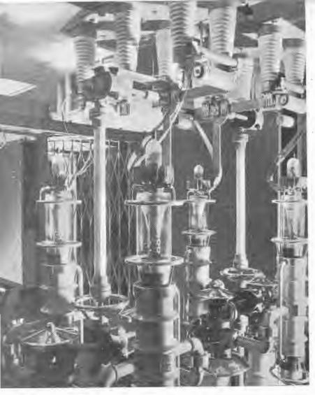
A 15,000 volt DC rectifier unit for use with the 100 kw. transmitter showing mer-cury vapour rectifier valves.
