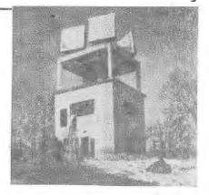
One of the seven microwave relay stations. A pair of shielded lens antennas provides two way transmission at 4000 Mc.
