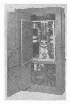
Side view of a 20 kw. H.F. Induction Heater, showing water-cooled oscillator valves and main tank coil.
