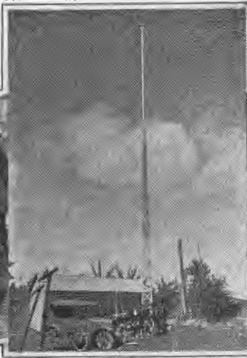
The lofty mast which supports 4ER's aerial system.
