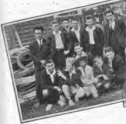
An informal snapshot of the members who helped with the renovating of the club rooms and the building of the transmitter and mast.
