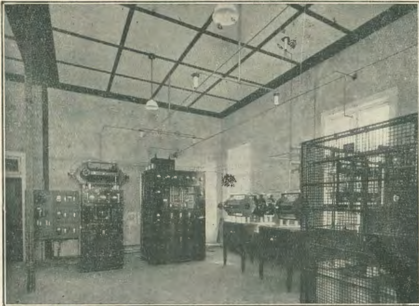
The Lower Half of the Transmitting Room at 4QG.
