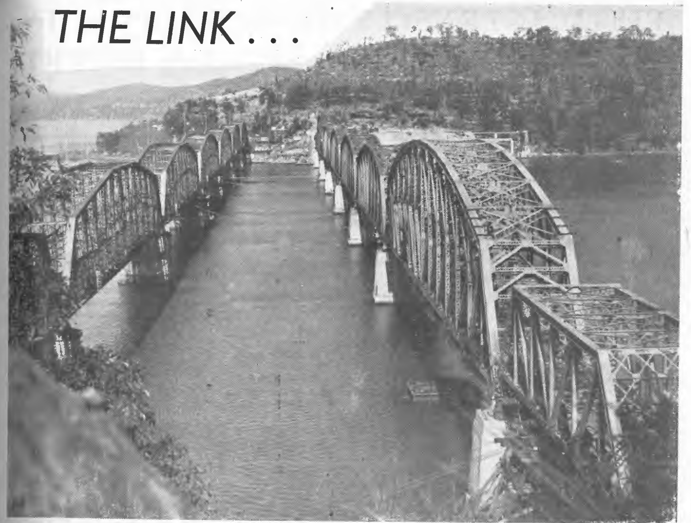
OLD AND NEW HAWKESBURY RIVER BRIDGES
