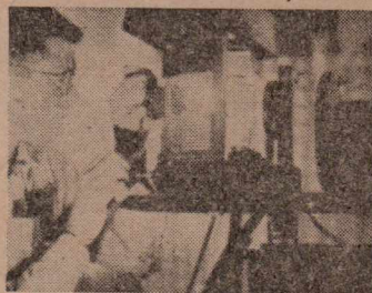
SPECTROGRAPH ... Analysis determines exact characteristics of metals to be joined.
