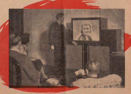
Mr. Baird's 600 line colour televisor. The screen receives either 600 line colour pictures or by pressing a button the B.B.C., 405 line monochrome pictures. It measures  $2^{\circ}6^{\circ}\times 2^{\circ}0^{\circ}$ . The set includes an automatic record-changing radiogram and an all-wave wireless receiver
