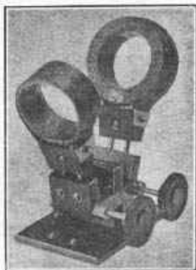
Fig. 1.—Honeycomb Coils in Use as Former.
