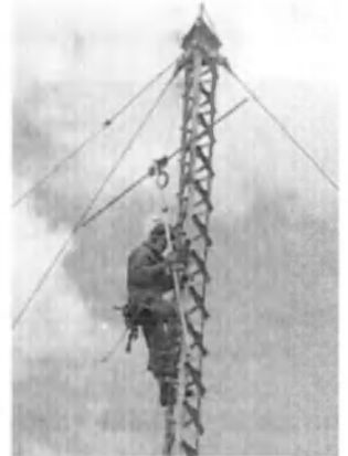
Roger VK7XRN, in harness, installing the 6m repeater receiving dipole on the Queen's Domain Clubroom's tower.
