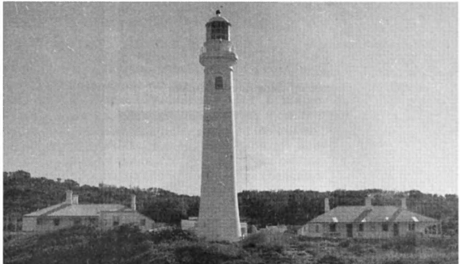
Point Hicks Lightstation: EGARC base was in the house on the right-hand side.
