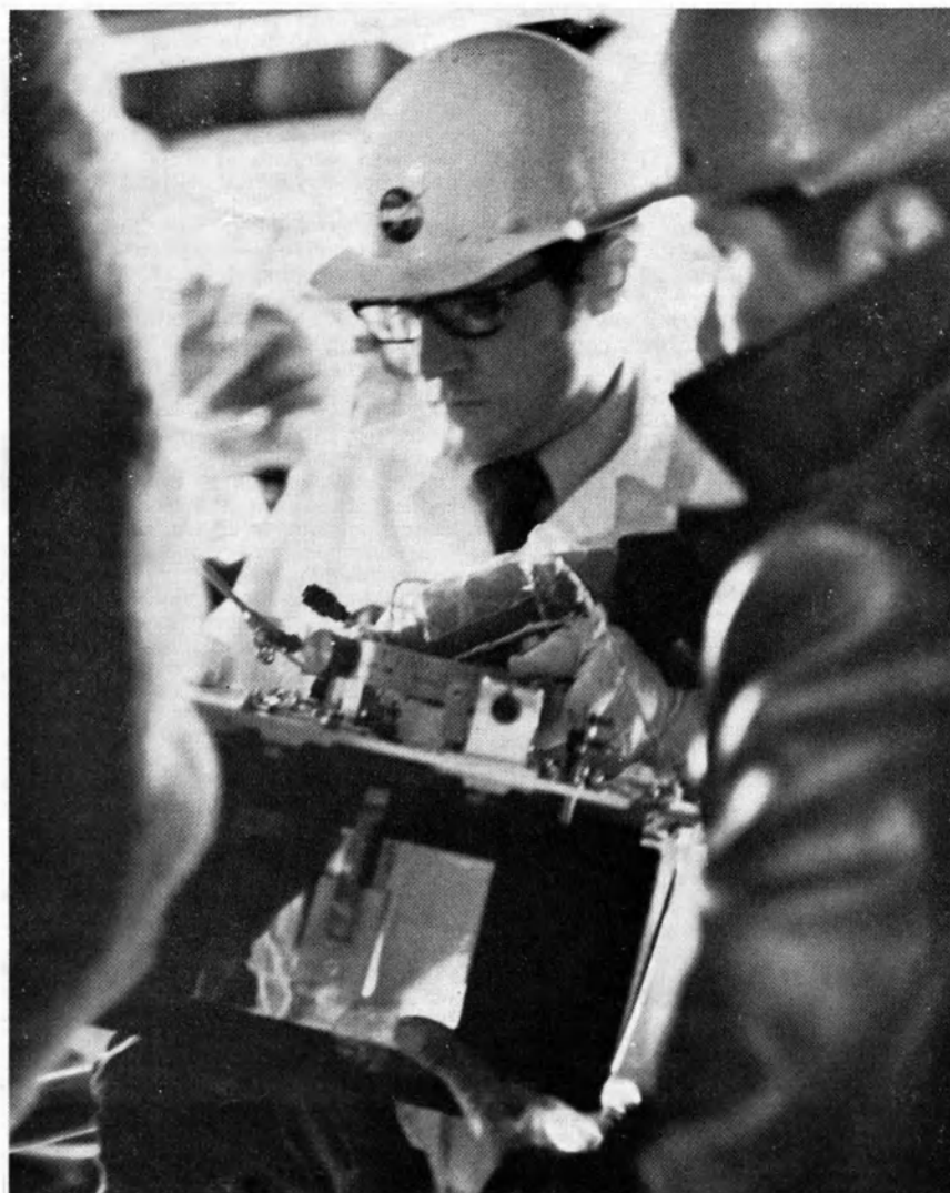
Jan King and assistant instal Oscar 5 Satellite in position on launch vehicle at fourth level of gantry, SLC 2 West, Vandenberg Air Force Base, Calif.
