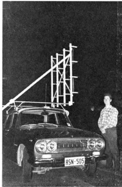
John VK5QZ with his roof-mounted 32 element 576 MHz. array.
