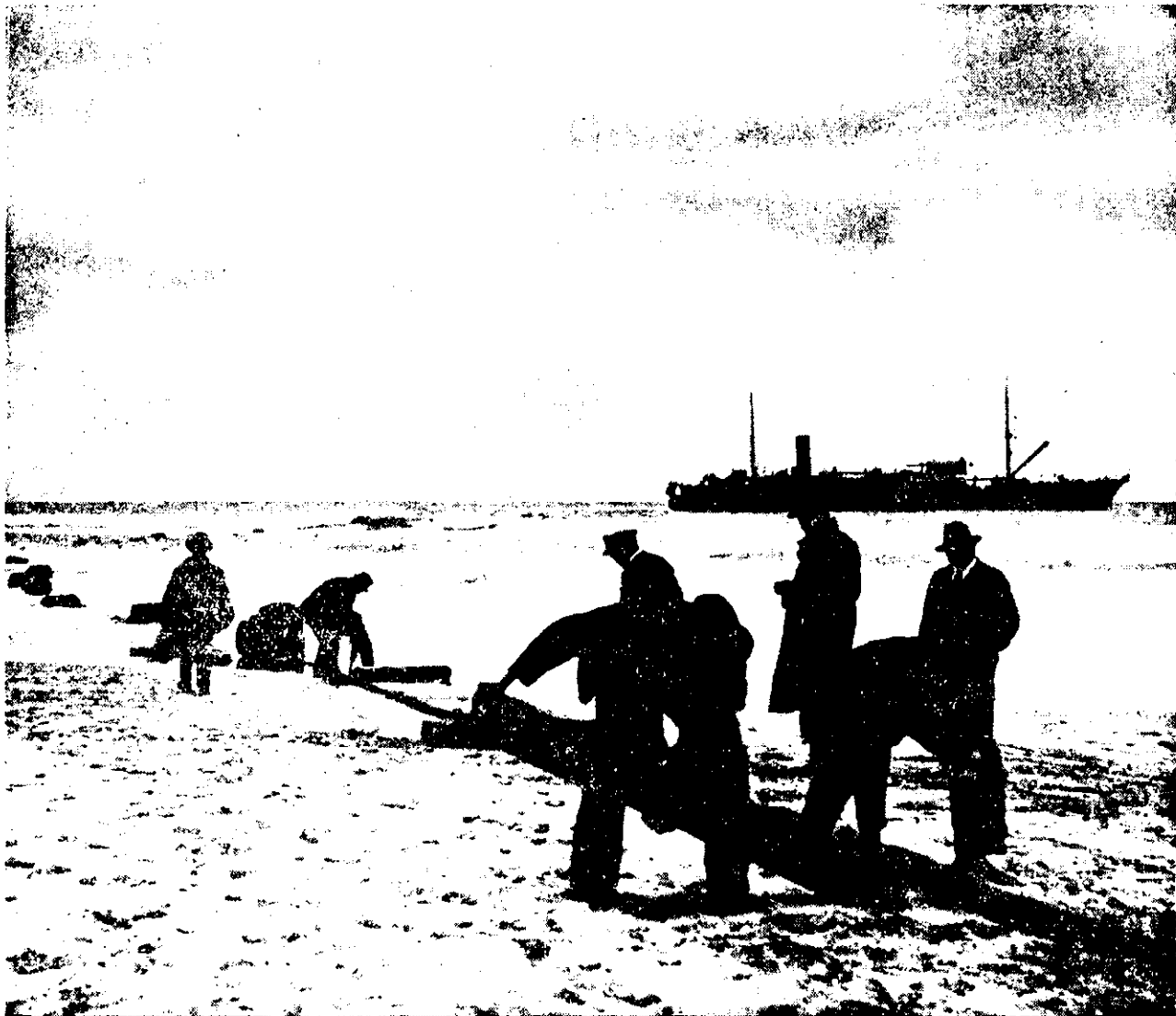
A P.M.G. team securing an underwater cable on the shore of Apollo Bay, Vic.
