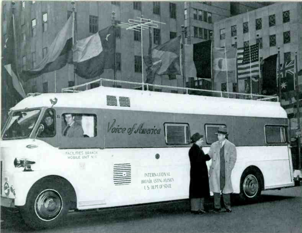
The "Voice of America" uses this RCA-equipped van to pick up and transmit remote programs.
