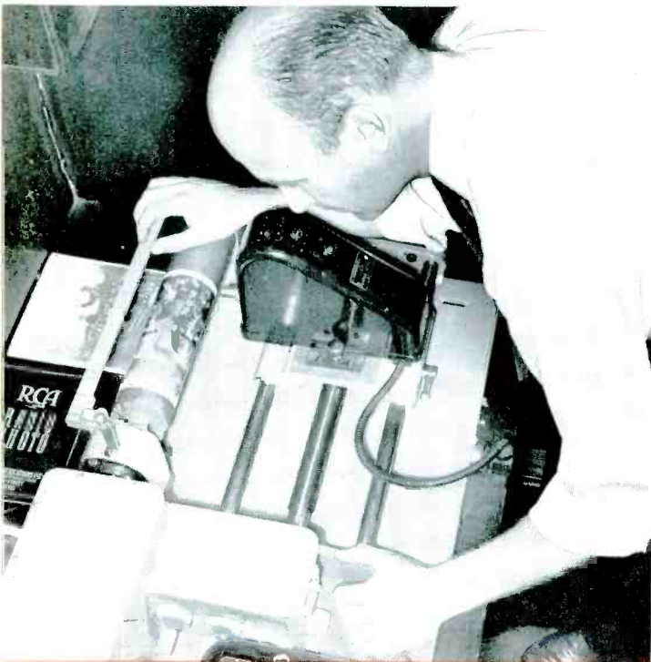
These radiophotos coming in on RCA's New York receiving cylinder have traveled 4,615 miles across the Great Circle route, through the air from Moscow.
