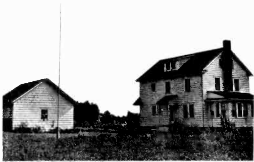
Figure 3—Home Installation with Pole Antenna and Underground Transmission Line
