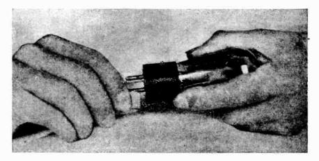
Figure 6-Method used to clean Radiotron prongs.
