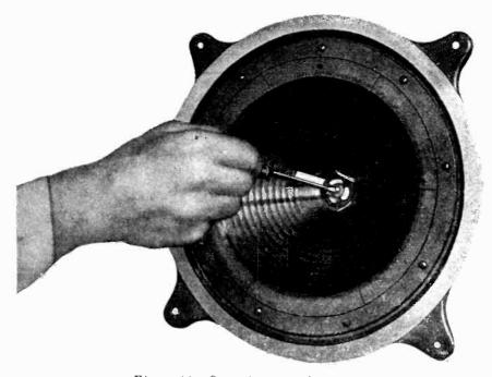
Figure 11—Centering reproducer cone
