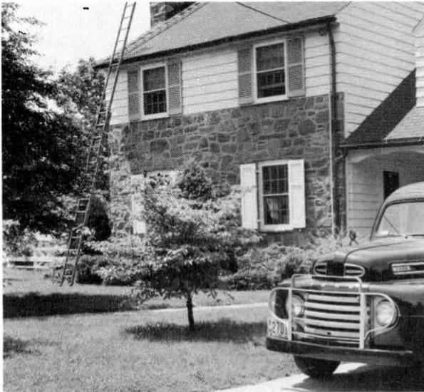
When a ladder is placed against a building, at least four rungs should extend above the point of contact with the building.
