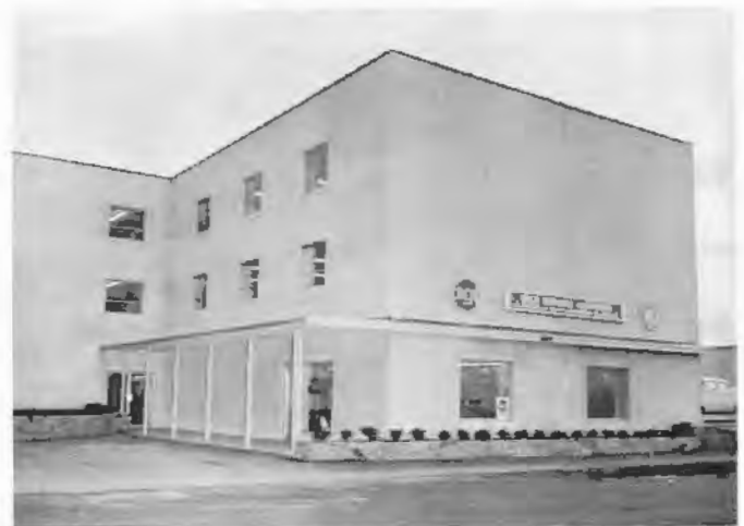
RCA Service Company, Riverton, New Jersey, headquarters for the construction of BMEWS in the far North
