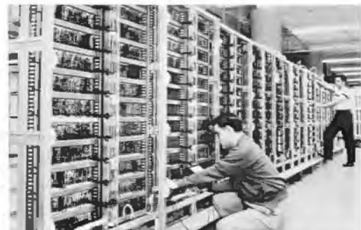
RCA-501 logic system, checked-out by IEP technicians at the Camden plant.
