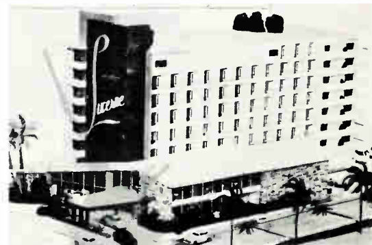
Miami Beach's new Lucerne Hotel, featuring RCA Antenaplex, Hi-Fidelity Sound & Intercom Systems
