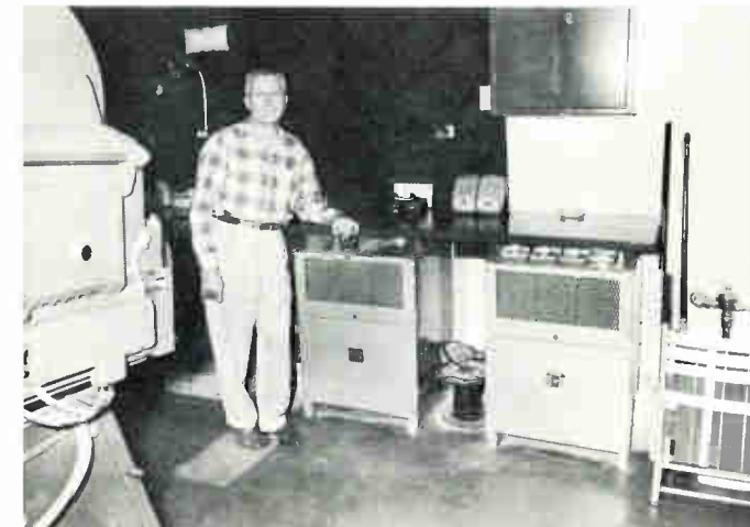
Engineer Rudy del Castillo surveys his completed work
