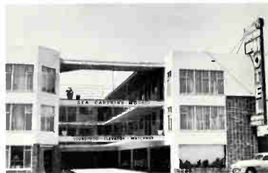
Sea Captain's Motel in San Francisco housing 37 RCA-TV receivers, plus protective service contracts
