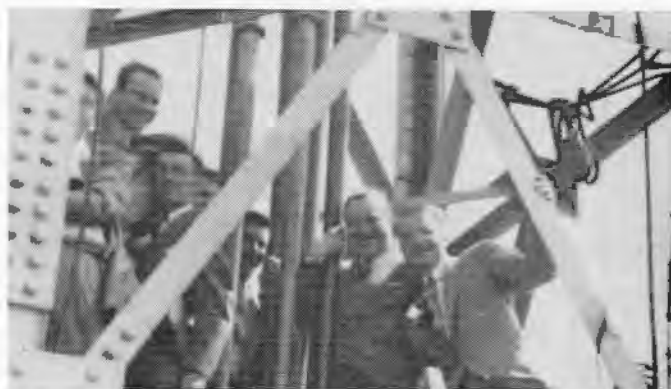
Toppers an top with top antenna atop Empire State Bldg.
