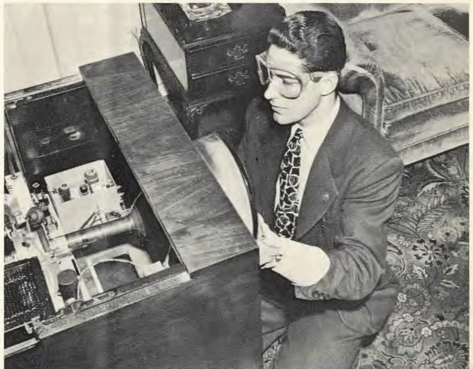
John Carter, TV Service Technician of Camden Branch, inserts a kinescope in the deflection yoke of the new 1949 TV model - BT244. He's using safety goggles and gloves similar to those soon to be distributed to TV branch personnel.
