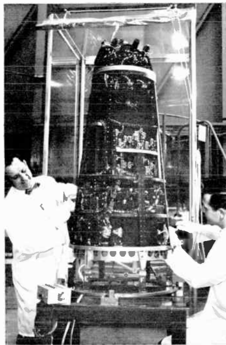
PASADENA—Field engineers Wilczynski and Nachbar test Ranger's TV system.
