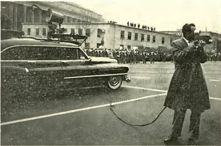
Fig. 7—Cadillac Telemobile Unit parked on Pennsylvania Avenue. The driver is operating the hand-held Vidicon camera.
