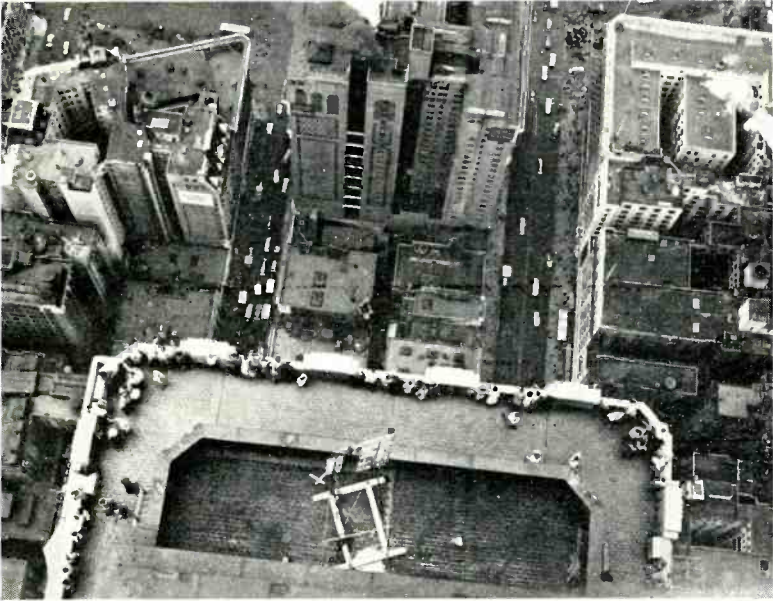
Fig. 8—The 510- and 910-megacycle antennas on the eighty-seventh floor balcony.
