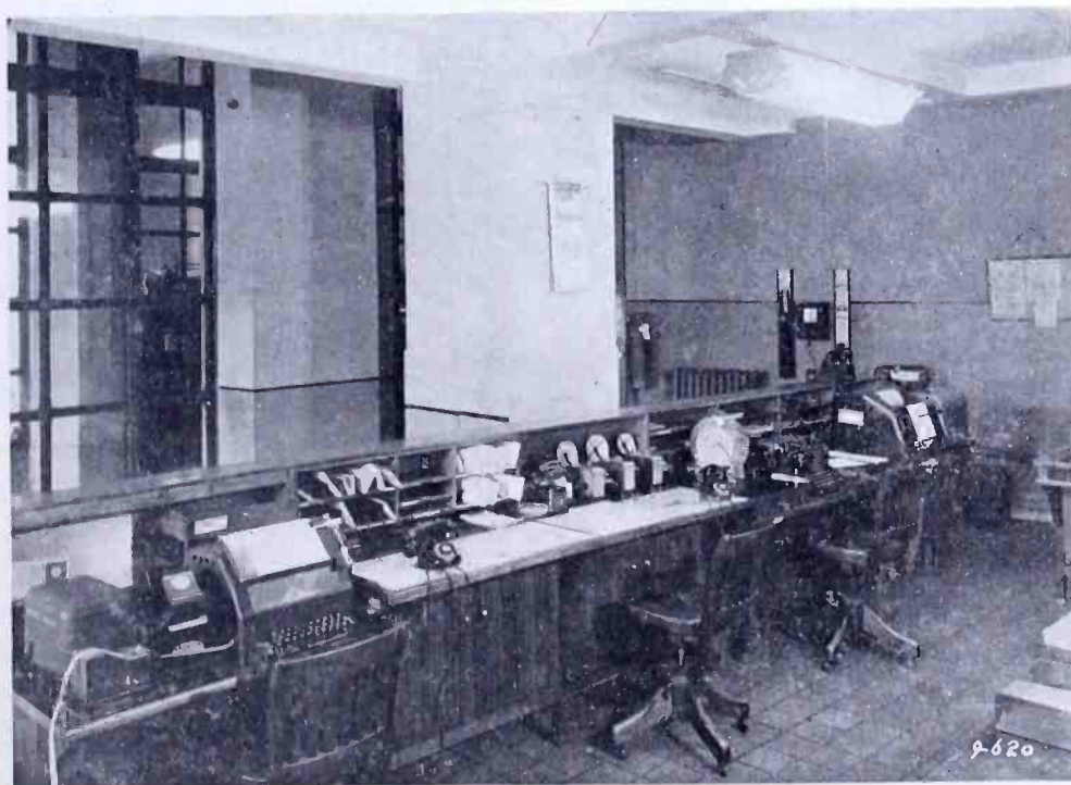
Fig. 9—A typical branch office installation. (The equipment for perforating and transmitting outgoing messages is shown on the left, and that for receiving incoming delivery copies on the right.)
