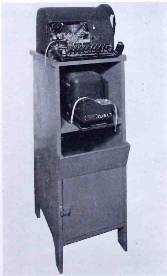
Fig. 16—Tape patching set.
