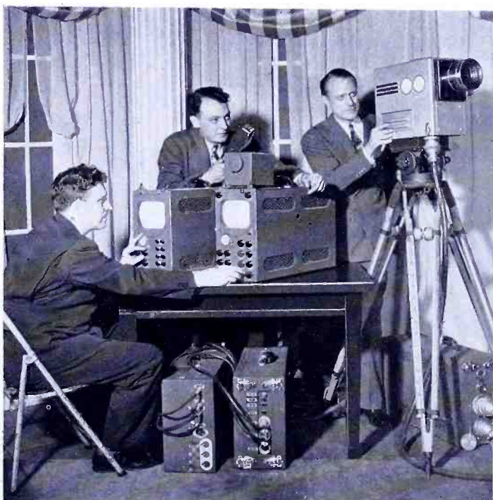
Fig. 4—Complete Single Camera Iconoscope Type Transportable Pickup Equipment.
