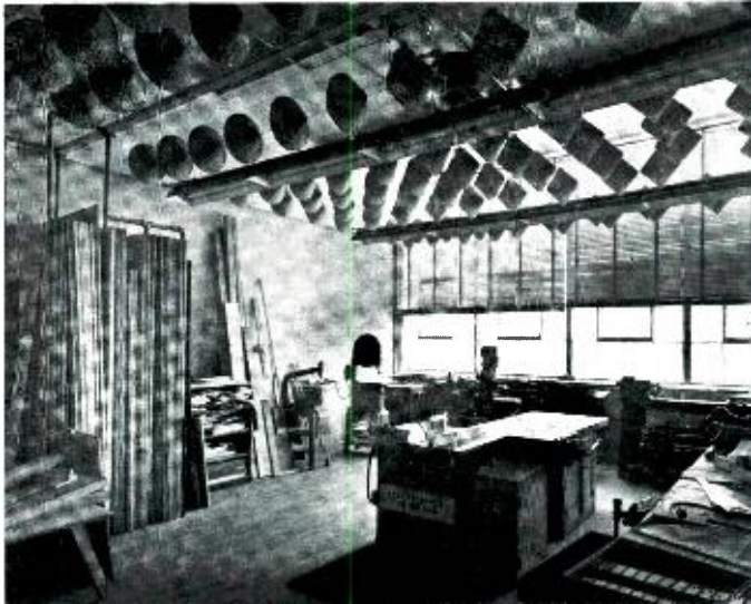
Fig. 20—Installation of the functional sound absorber in the cabinet shop.
