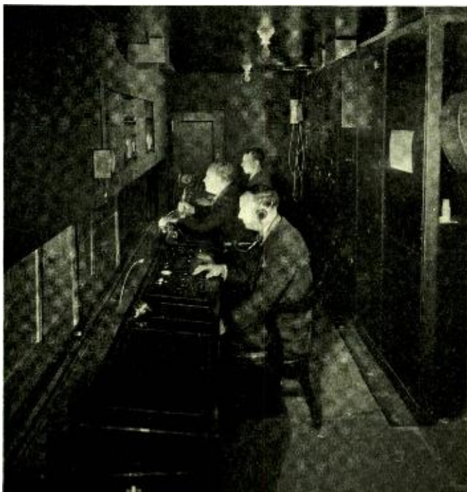
Fig. 4—Television studio control room
