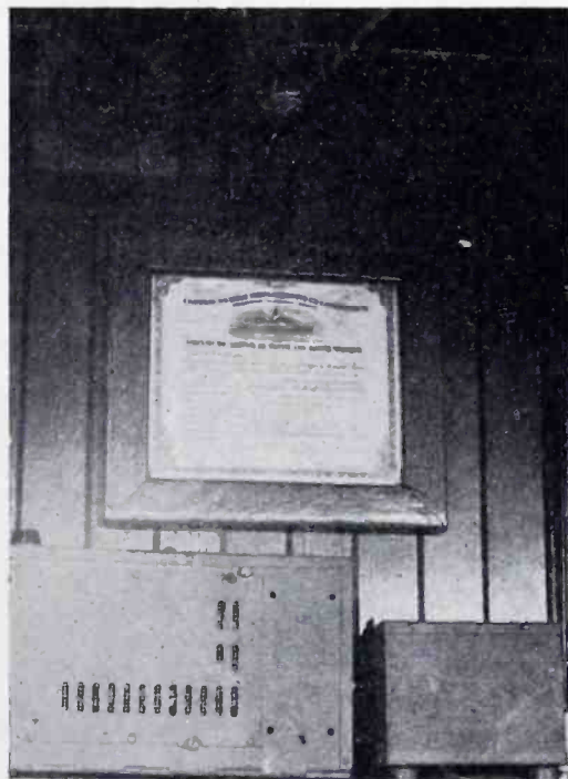
Fig. 2—Tugboat receiver installation.
