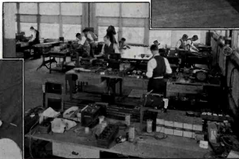
Shielded Test Room, for making sensitivity and selectivity radio-frequency tests
