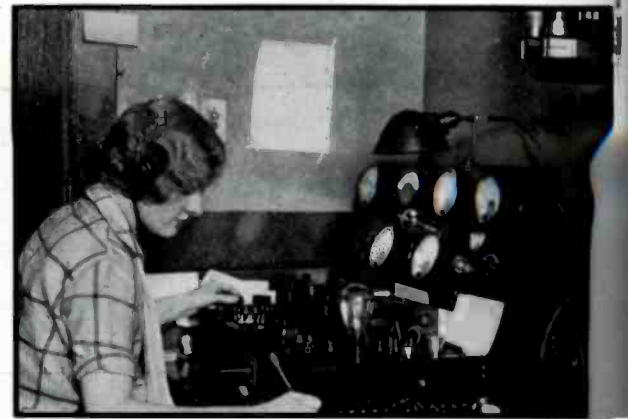
Checking the electrical characteristic of RCA Radiotrons goes on every day
