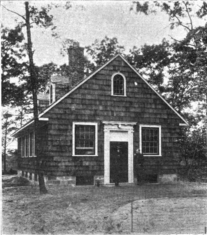
RIVERHEAD RECEIVING STATION
