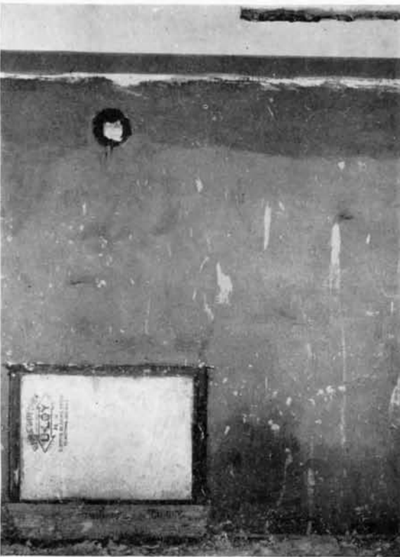
Figure 10. Rough plaster surface ready for acoustical treatment.
