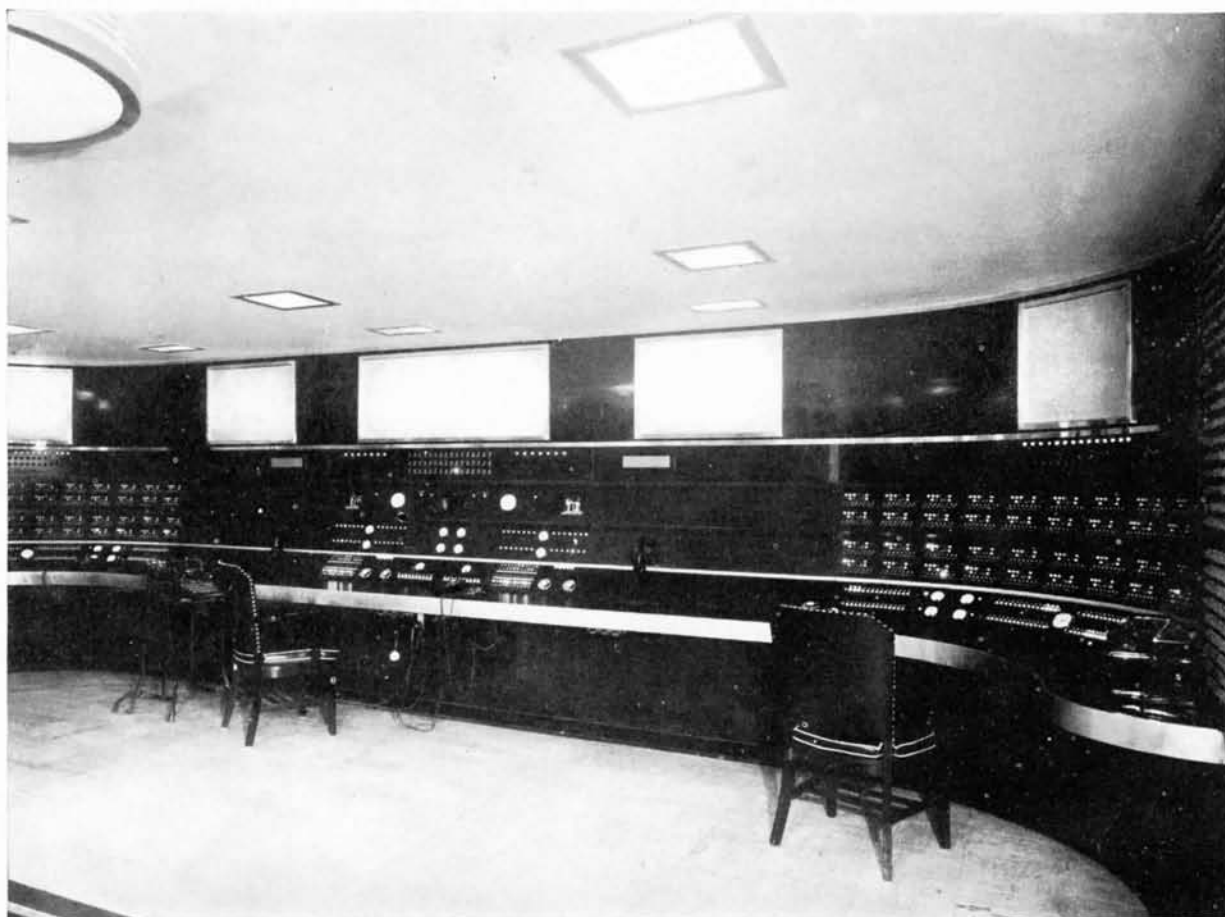
Figure 27. The master control desk, the "nerve center" of broadcast activities at Radio City. The left and right sections of this desk are duplicates, the middle section is supervisory in function. On the panel near the ceiling may be seen the loudspeaker openings.
