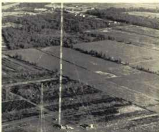
BOUND BROOK —From Radio City, operators send program out by wire to broadcasting transmitters of NBC's 137 stations on Red and Blue Networks. Typical is WJZ, at Bound Brook, N. J., showing 640-ft. antenna designed by RCA Victor engineers at Camden, N. J.
