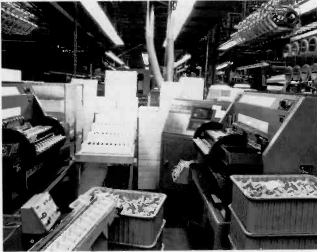
Production winders for ROSE transformer primary coils in operation at CE's component plant in Indianapolis.
