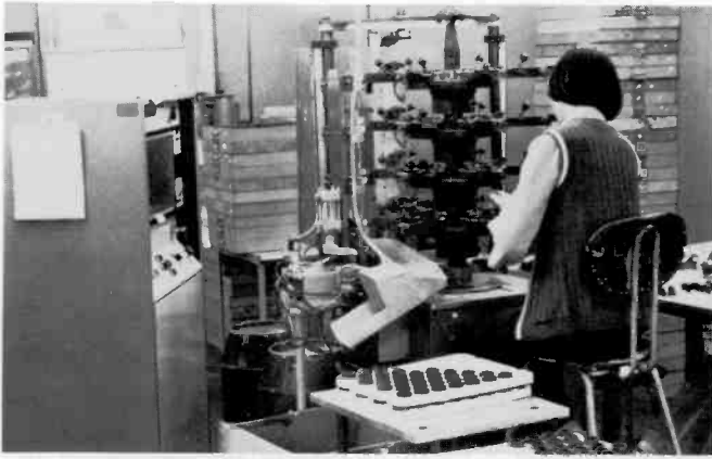
Fig. 1. Numerically controlled yoke winding for black and white TV receivers.
