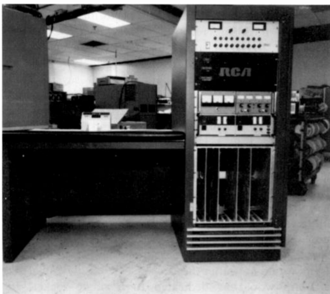
Fig. 1. GALT V switching-time console (with door removed).
