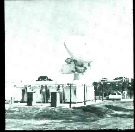
AN/TPQ-18 , the transportable version of the FPQ-6, is shown set up on transportable shelters.
