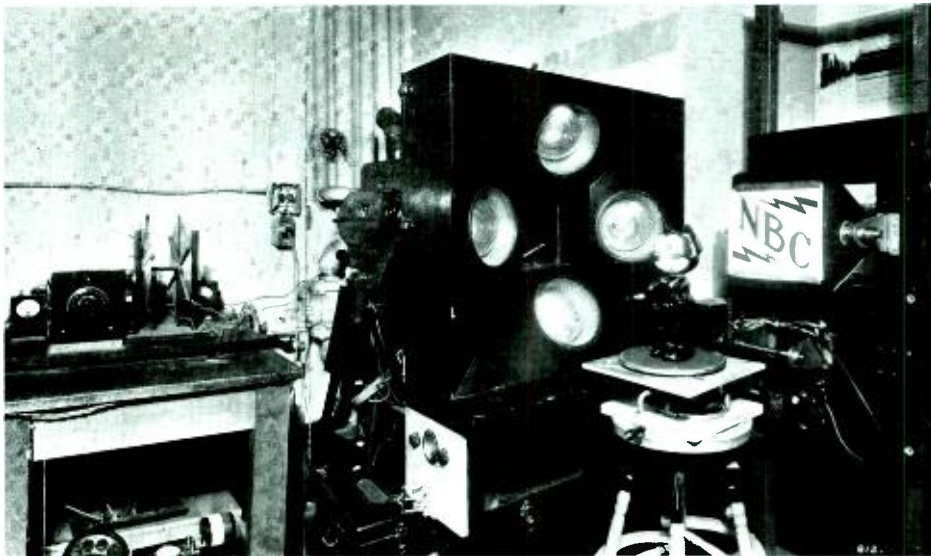
11 The first television camera used a 48-line mechanical scanning disc with four photocells for light pickup. Experimental station W2XBS was located at Van Cortland Park, New York. 12 The first television star, Felix the Cat. Felix was bathed in high-intensity carbon-arc light and rotated on a turntable to demonstrate tv's motion-capturing ability. The image was barely the size of a playing card. 13 The first NBC television logo.
