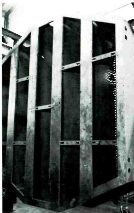
Fig. 18—The structure ready for assembly. Note the four main vertical flanges of the antenna structure.
