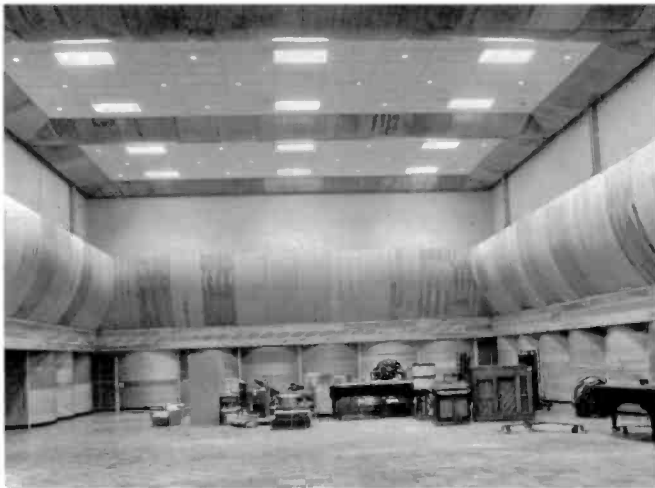
Fig. 6—Looking toward the wall opposite the platform in Studio A showing the ceiling sections raised to full height. Each of the three main ceiling sections has six fixtures distributed over the middle or absorptive area (0.8 coefficient) and a perimeter consisting of reflective convex wood panelling 4 ft. wide (0.2 coefficient). This illustration also gives a better view of the 8-ft-high horizontal convex plywood panelling covering the middle section of the walls. This horizontal panelling is hinged at the lower edge and may be lowered in individual 8-ft-wide sections by means of manually operated winches.
