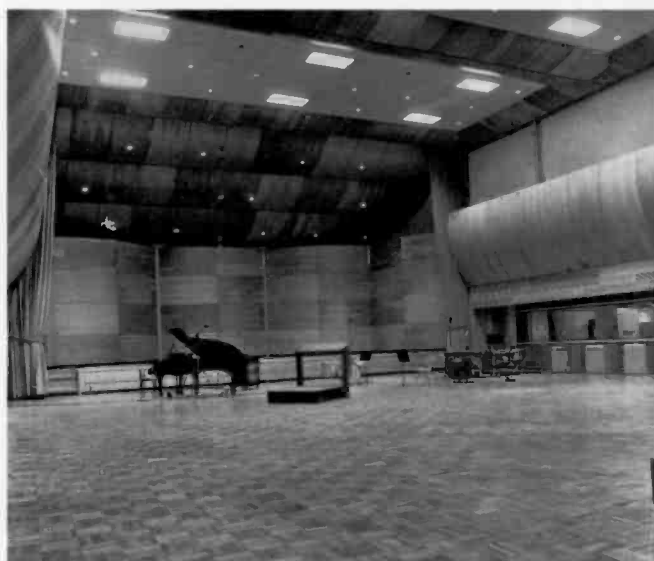
Fig. 3—The platform end of Studio A, showing the convex wood panels of the stage ceiling and walls in a "flared" position to form an orchestra or choir shell. Note that the ceiling in the studio proper is raised to full height, approximately 10 ft. above the side-wall horizontal convex wood panelling. Under the wood panelling is the control room window which is convex to match the wall treatment contour.
