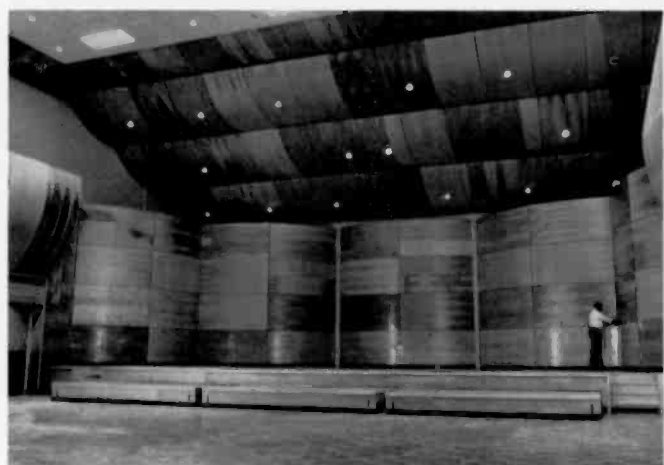
Fig. 4—Closeup view of the platform shell with wood panels in "flared out" position.
