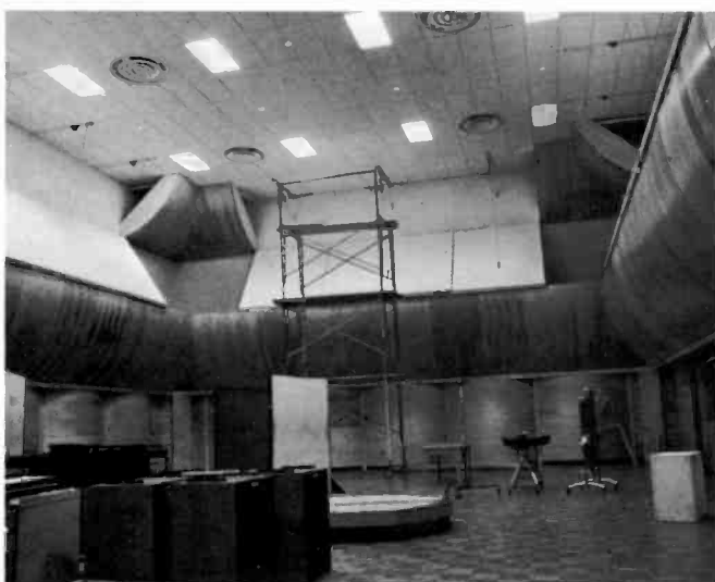
Fig. 14—General view of the studio with the uppermost hinged ceiling corner panels lowered, completely exposing the absorptive backside of the panels.
