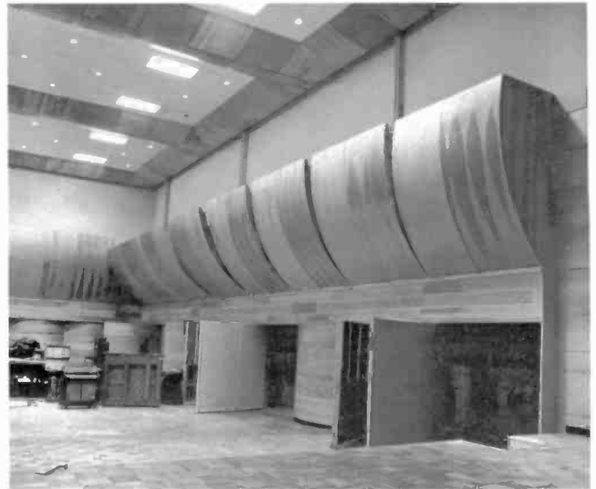
Fig. 7—The three types of adjustable acoustical elements in the main portion of Studio A: the lower hinged vertical wainscot panels for separating the direct sound sources and for controlling the local environment around them; the middle hinged horizontal wall panels for controlling the first or early reflections; and the movable ceiling sections for controlling the later diffuse reverberations.
