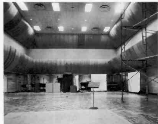
Fig. 13—View of Studio B showing the three types of adjustable acoustical elements used: the lower hinged verticle wainscot panels, similar to panels used in Studio A for the purpose of separating the direct sound sources; the middle hinged, horizontal wall panels, also similar to panels used in Studio A for controlling the first or early reflections; and the uppermost hinged wall panels at the ceiling junctures for controlling the later diffuse reverberations. Also shown is the suspended ceiling of glass-cloth-faced fiberglass panels (absorption coefficient is 0.8).
