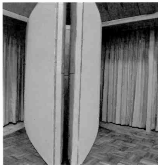
Fig. 17—Closeup of two wainscot panels opened in one corner.
