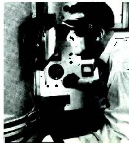
Fig. 3—F. P. Chiovarou operating electron-beam evaporator used in production of thin-film capacitors.
