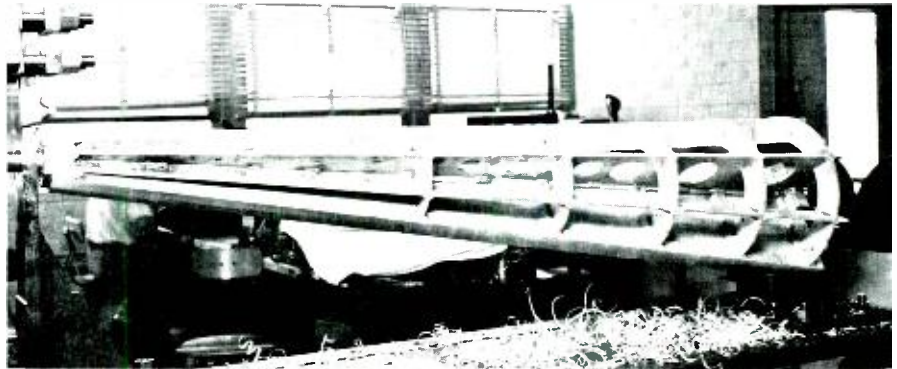
Fig. 6—Revolving cone during fabrication.
