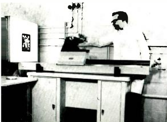
Fig. 6—D. W. Mann Reticle Camera used for making the precision reticle.
