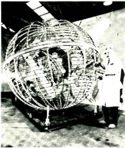
Fig. 2—Magnetic Tests of TIROS II.
