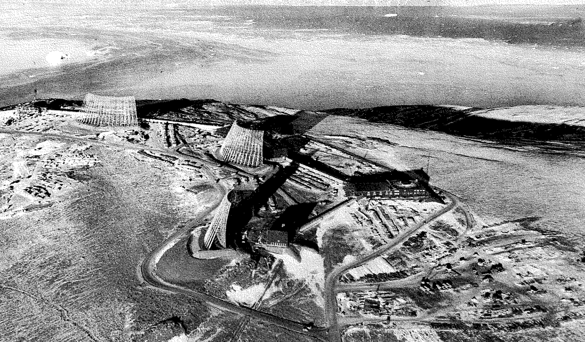
Fig. 1—This aerial view at one of the Sites shows much of the technical complex. Shown are scanner and radar transmitter and computer buildings in addition to the huge antennas. The antennas are larger than a football field.
