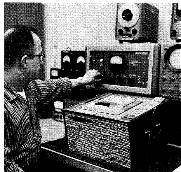
Fig. 12—A. J. Curry, Quality Control Inspector is shown operating a laboratory test setup for making Quality Control checks on the completed tape recorder instrument.
