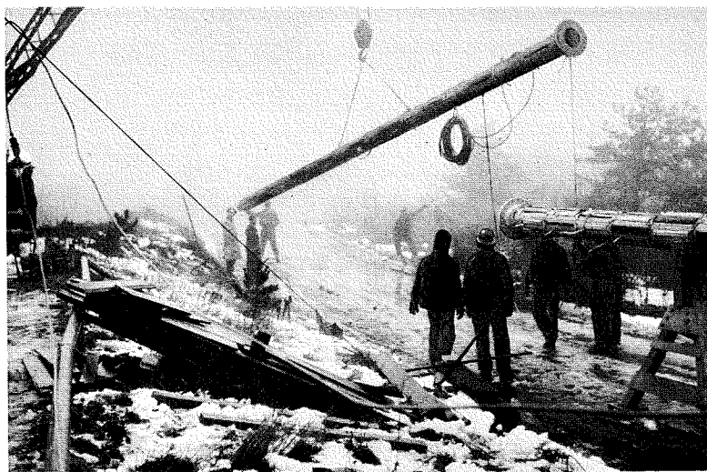
Fig. 16—View at Wilkes-Barre, Pa., showing the placement of the high-gain antenna on "horses" for ground checkouts.
