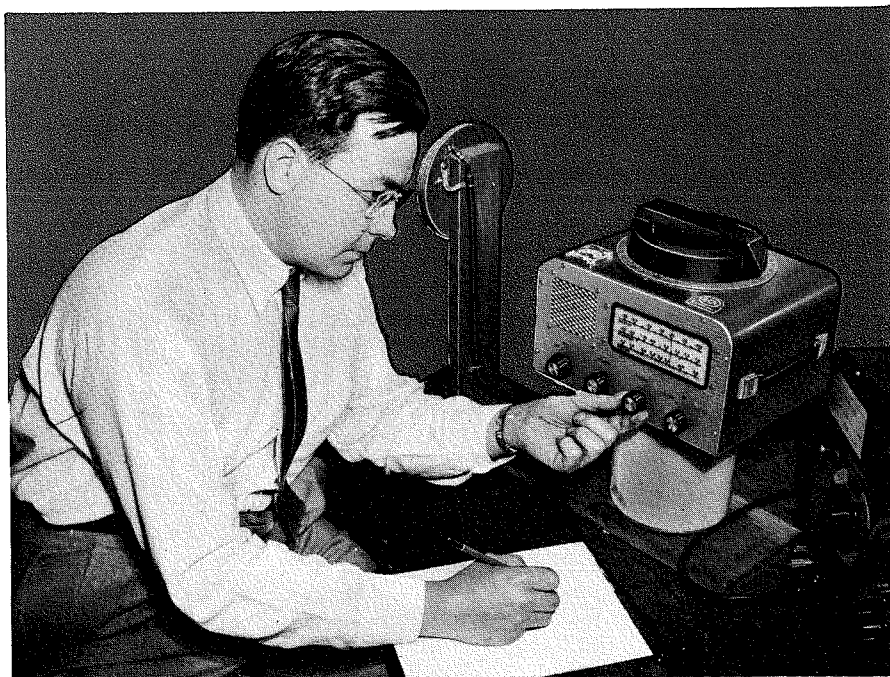
Fig. 4—Walter S. Glazar, associate project engineer, taking sensitivity measurements, using a transmitting loop.
