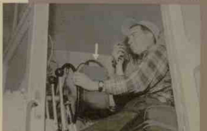
Fig. 18—Radio transmitter-receiver unit is installed inside cab of road grader.
