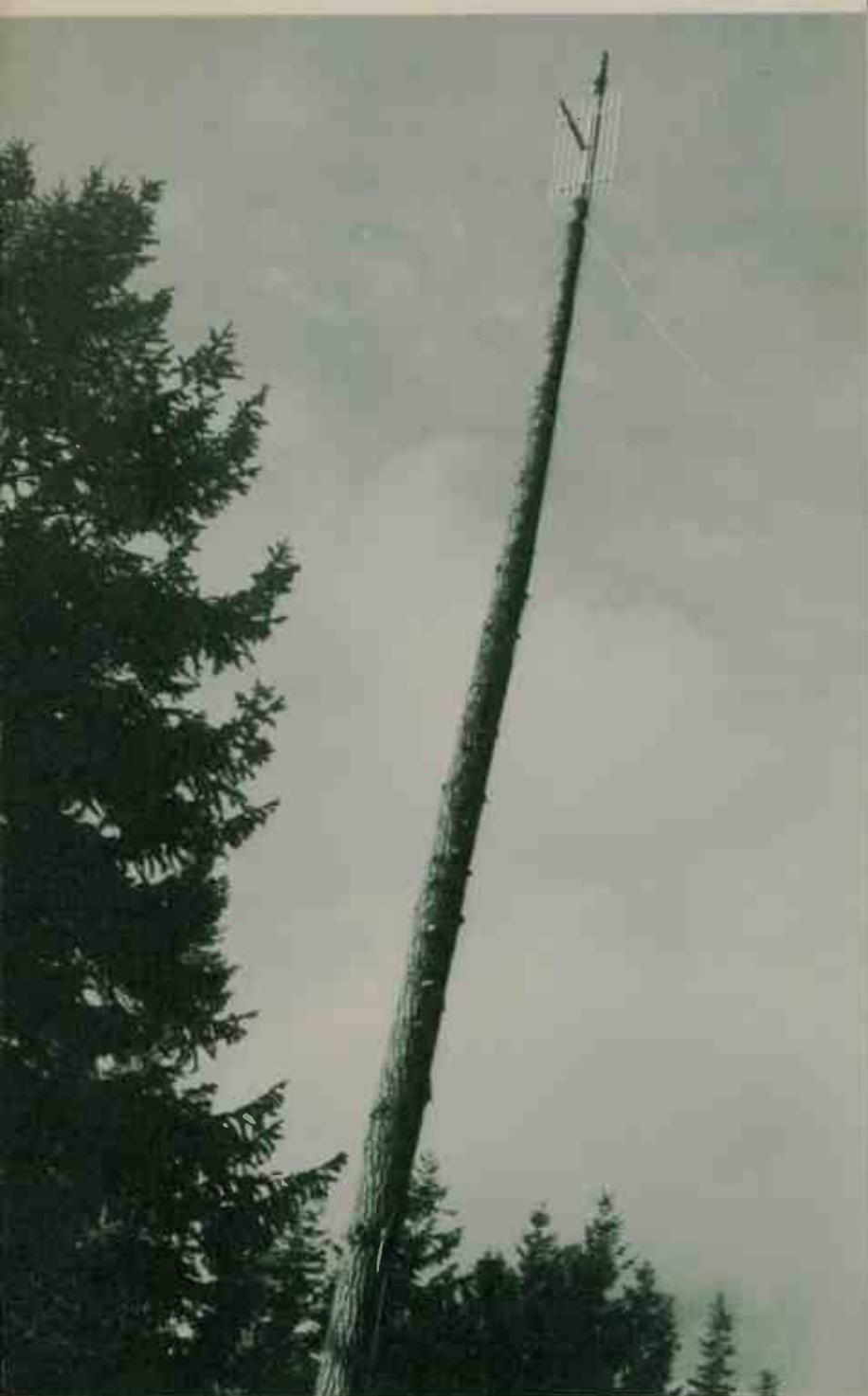
Fig. 8—At Copper Mountain 152-mc directional antenna is oriented to Allison Pass.
