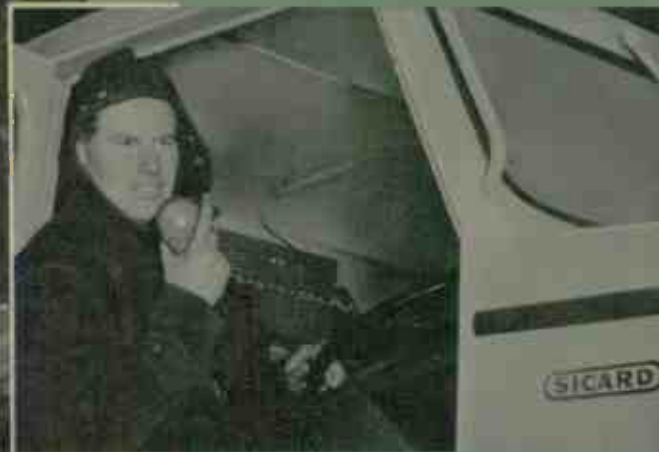
Fig. 11—Operator of snow blower keeps in touch with highway office by Carfone radio.
