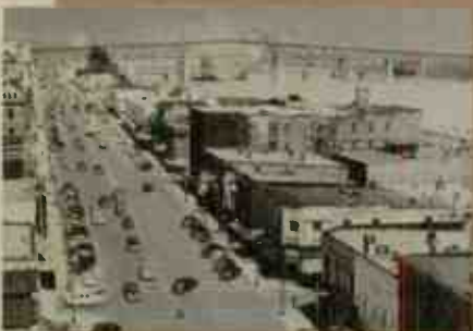
Fig. 5—New Westminster is protected by Carfone radio in police and fire vehicles.
