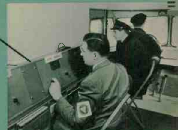
Fig. 9—Control room accommodates crew of eight.
