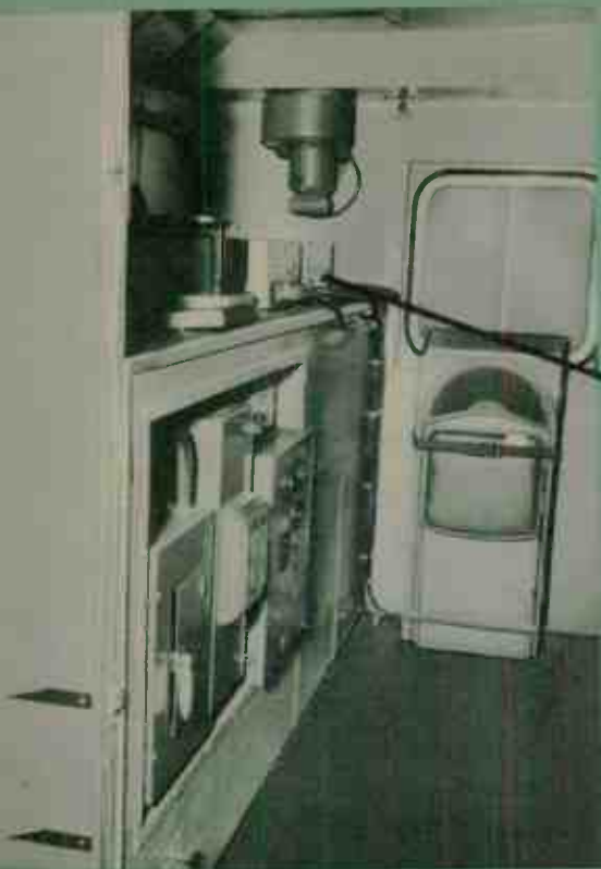
Fig. 3—Rear of van contains emergency generator, controls, and mobile transmitters.
