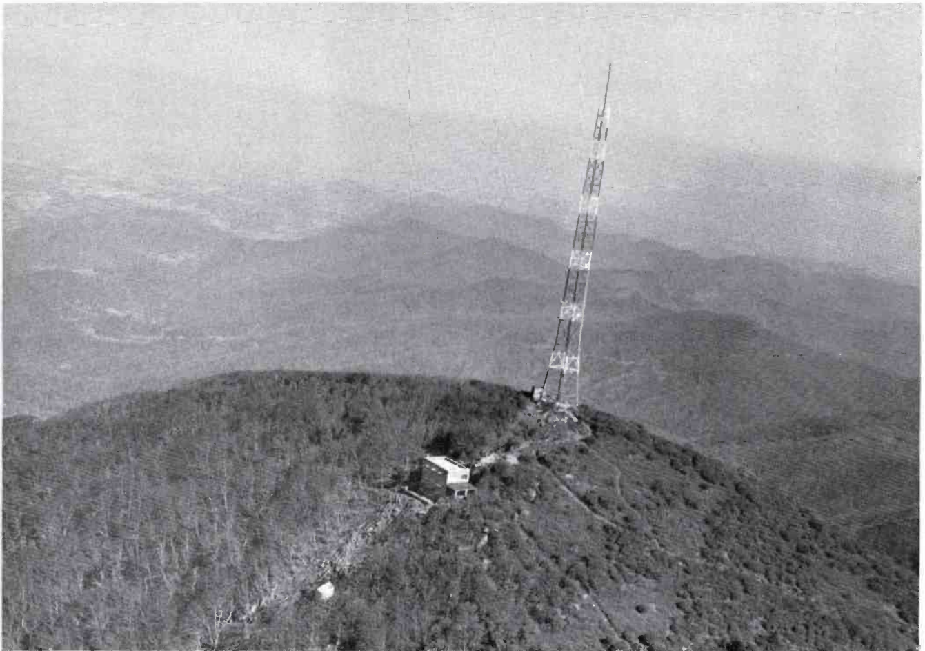
FIG. 1. Aerial view of the WLOS-TV transmitter site atop Mt. Pisgah shows rugged terrain. Transmitter building is structure located in the foreground. Studios are located off to the left about 18 airline miles away in residential area of Asheville, N. C.
