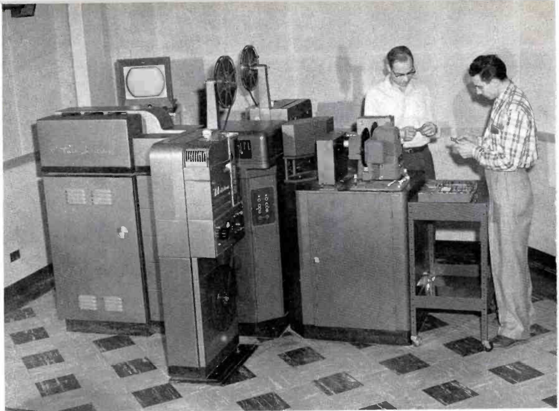
FIG. 21. This station has the first RCA 3-vidicon color film system employing the new TP-15 Universal Multiplexer.
