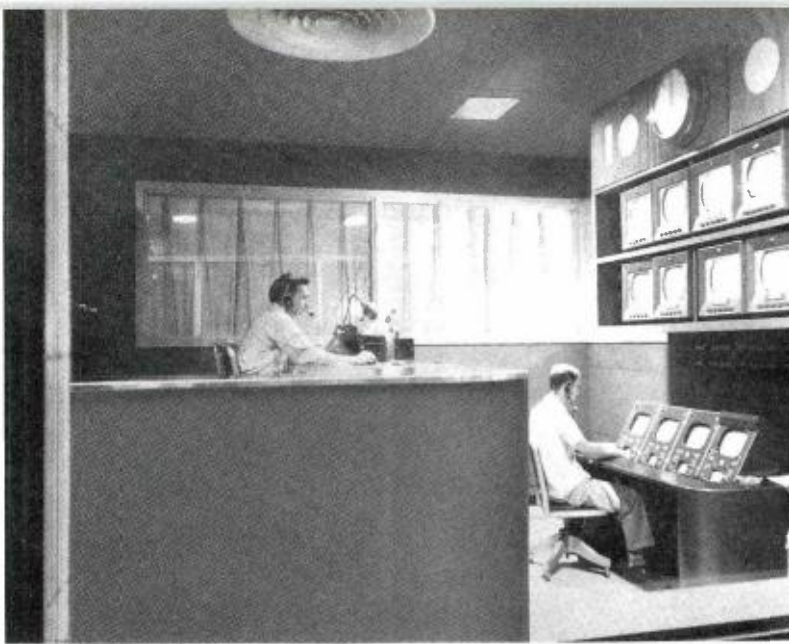
FIG. 19. Studio control room contains two levels. Upper level contains audio and video switching.
