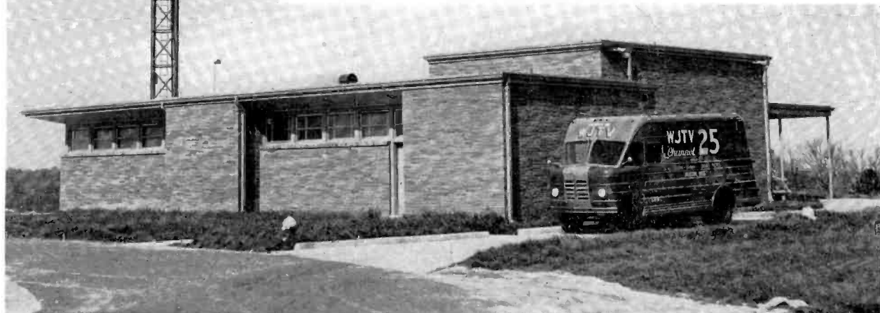
FIG. 1 (below). Exterior view of the WJTV Brick Transmitter Building and Tower.
