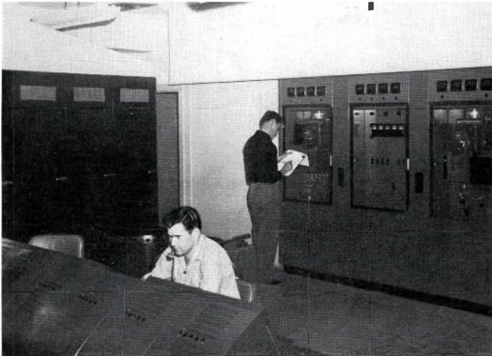
FIG. 11. View of the WJTV transmitter room showing the RCA TTU-1B, 1 KW UHF transmitter and partial view of the console. Note that provision is made for addition of RCA high power amplifier. Harold Townsend is shown at the transmitter and R. K. Somers at the console.
