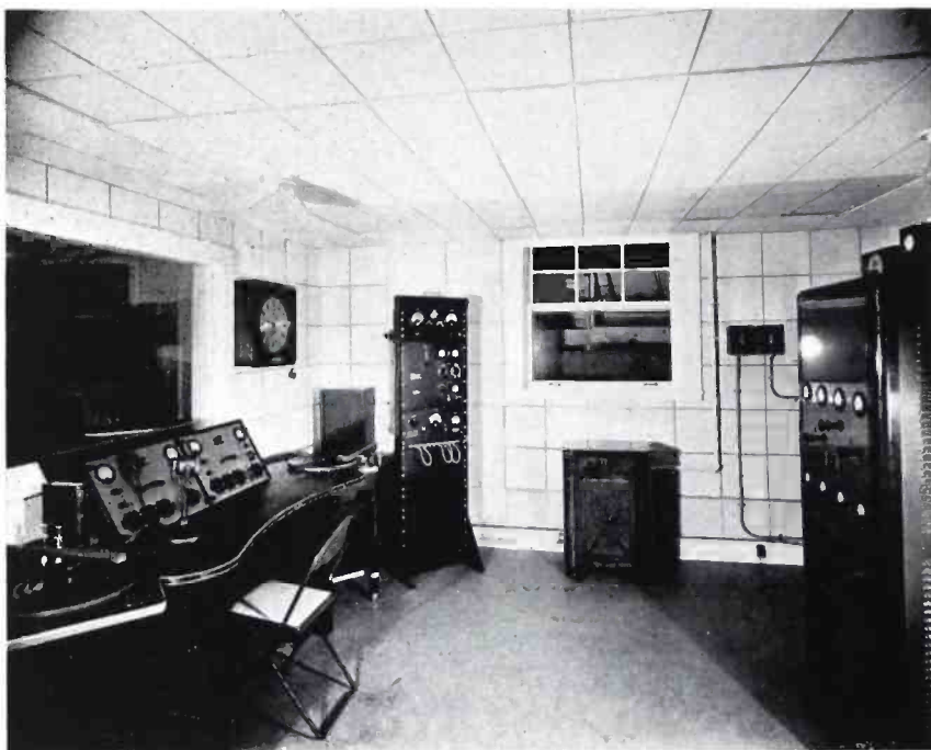
The RCA Equipped Control Room at KBND.
