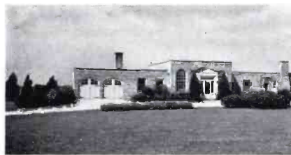
WMBI Transmitter Station at Addison, Ill.
